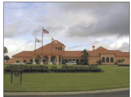
Extensive coordination with the Bear Lakes Country Club minimized disruptions to the golf course during lining operations.
