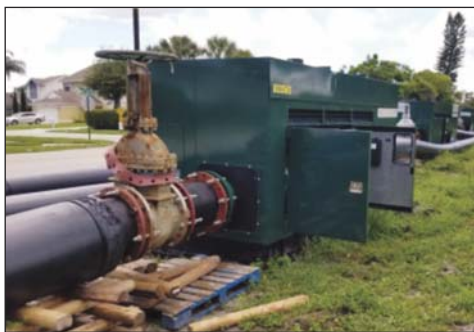
Bypass pumping through three 24-in. HDPE pipes was required to deliver 30 mgd to the treatment plant during lining operations.
