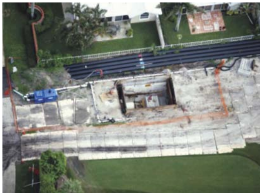
Bypass piping and liner insertion pits were located to limit impacts on the property.
