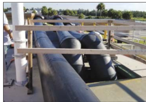
Bypassed flows were discharged directly into the headworks structure.
