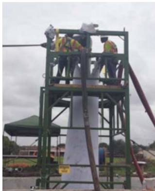
The wetted liner tube was positioned vertically over the insertion pit (left) and inverted into the open end of the force main (right).
