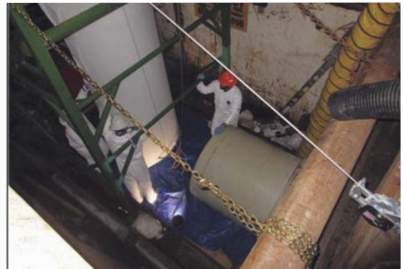
The wetted liner tube was positioned vertically over the insertion pit (left) and inverted into the open end of the force main (right).
